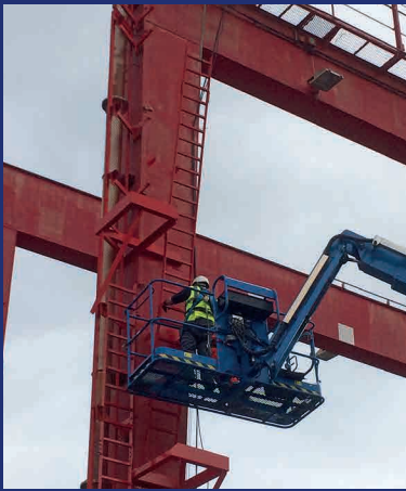
Safety enhancements at Bristol Port
